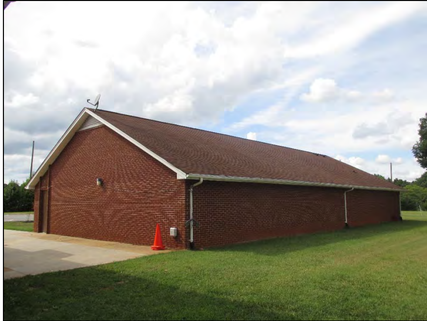
Figure 17: Center Baptist Church, facing northwest to side-gabled outbuilding
