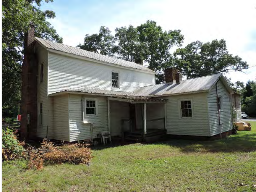
Figure 50: Suggs House, facing southwest to rear elevation
