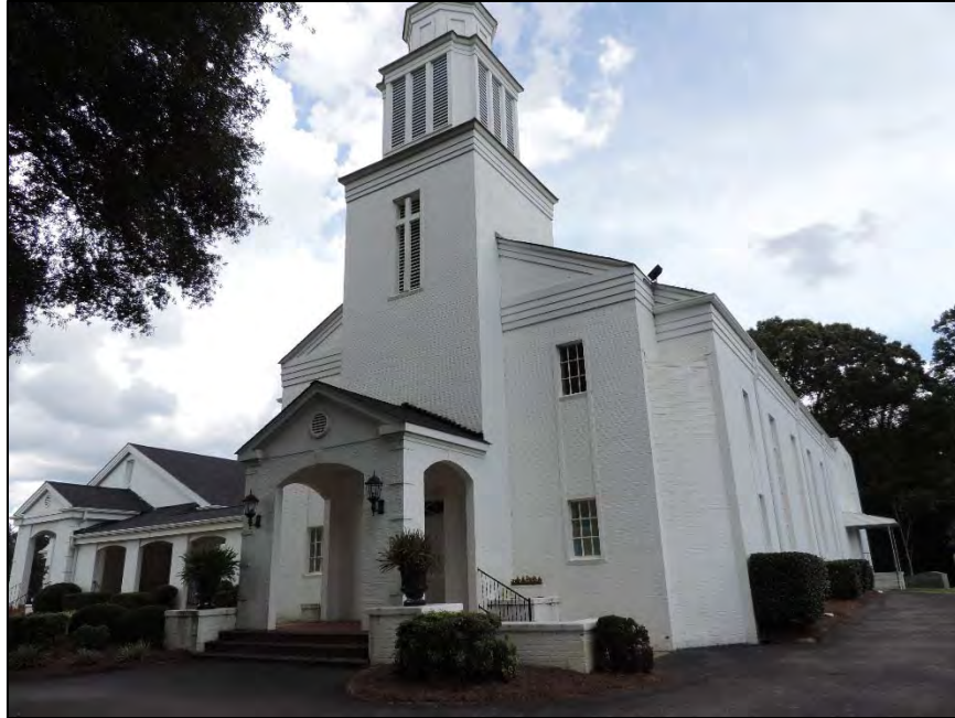
Figure 65: Facing northeast to New Hope Presbyterian Church
