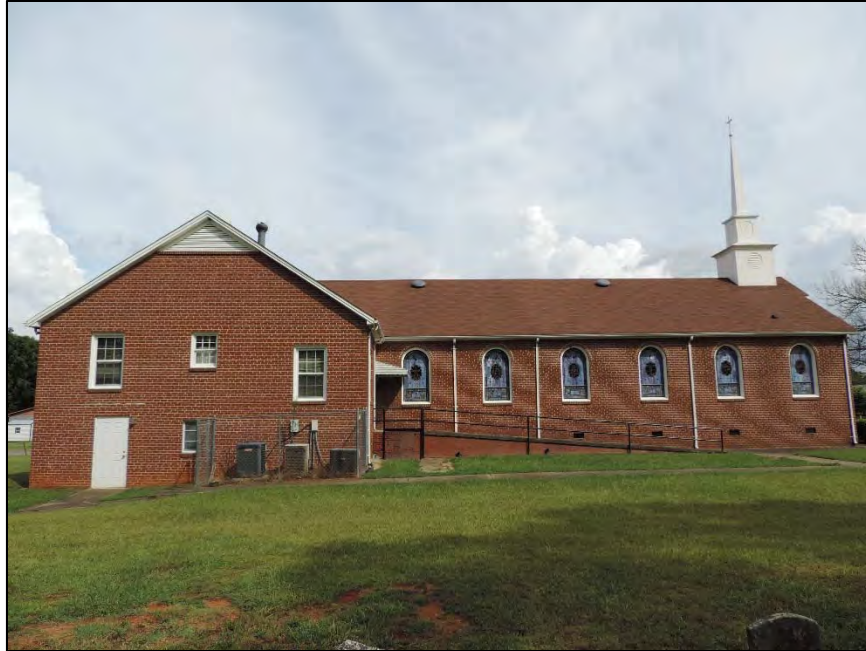
Figure 30: Neely's Grove Church, facing southeast to northwest side elevation
