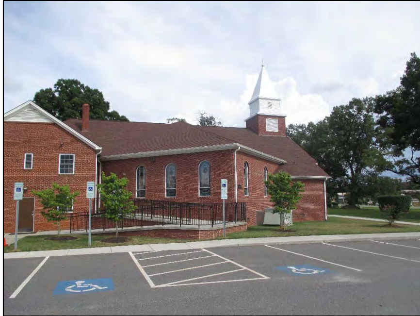
Figure 11: Center Baptist Church, facing southeast to side elevation
