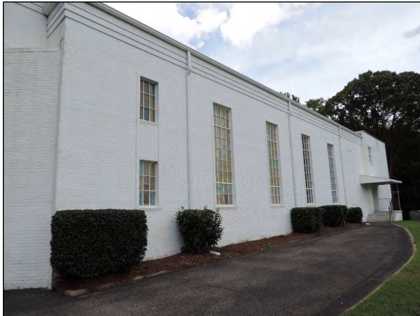
Figure 68: New Hope Presbyterian Church, facing northeast to south side elevation
