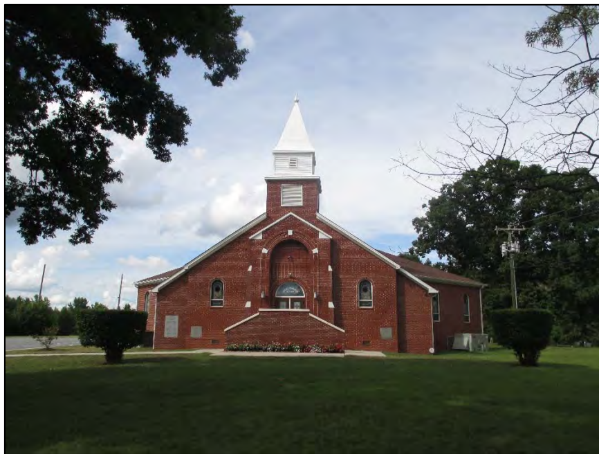
Figure 7: Facing northeast to Center Baptist Church
