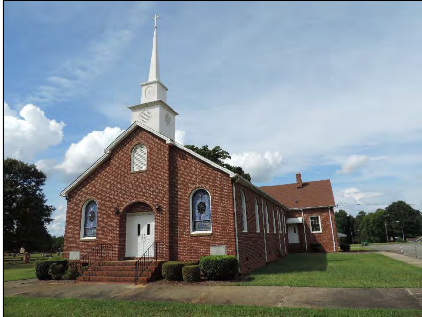
Figure 27: Facing north to Neely's Grove Church
