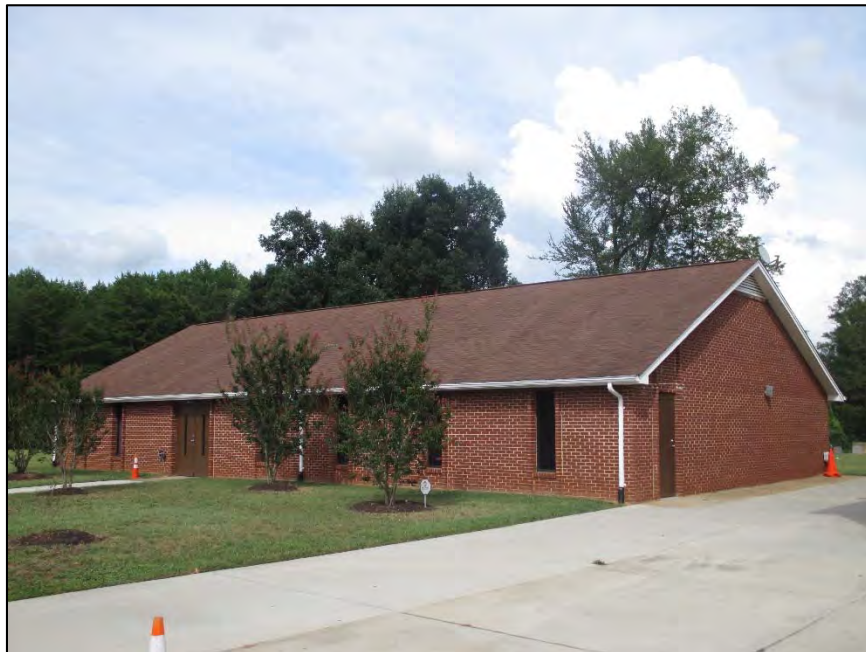
Figure 16: Center Baptist Church, facing northeast to side-gabled outbuilding
