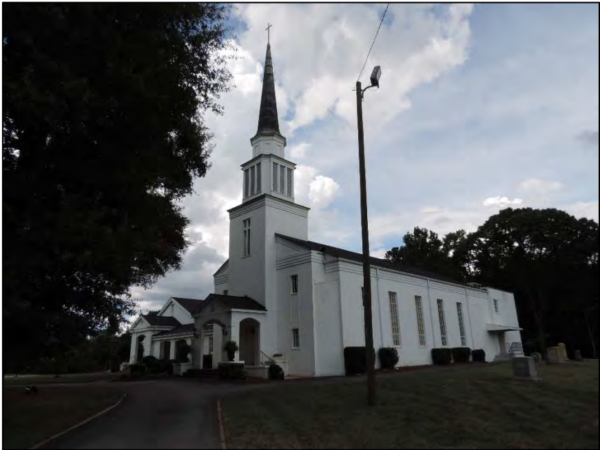
Figure 64: Facing northeast to New Hope Presbyterian Church
