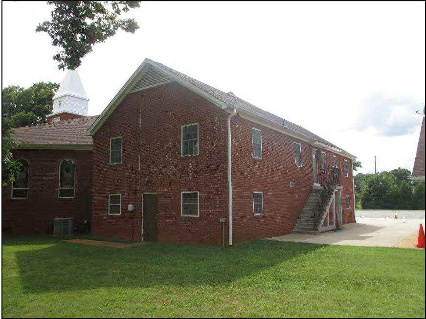
Figure 13: Center Baptist Church, facing southwest to rear wing
