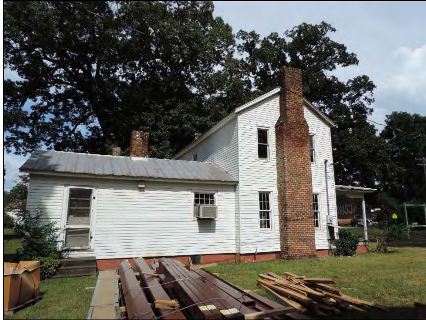
Figure 49: Suggs House, facing southeast to west side elevation
