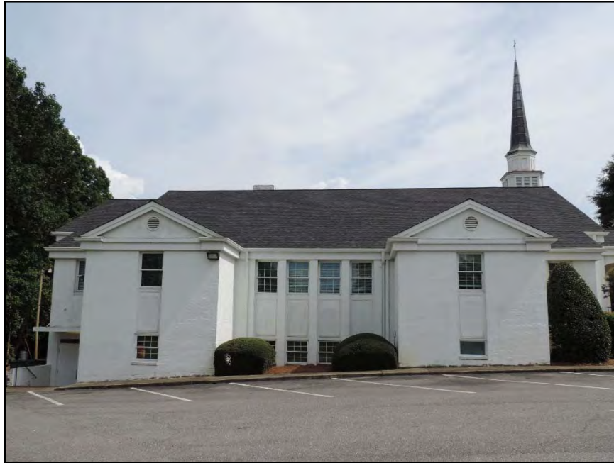
Figure 77: New Hope Presbyterian Church, facing southeast to north side elevation of Education Building
