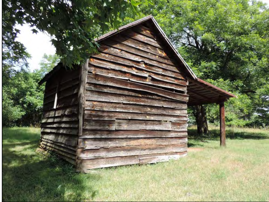
Figure 57: Suggs House, facing southeast to outbuilding located to rear of house
