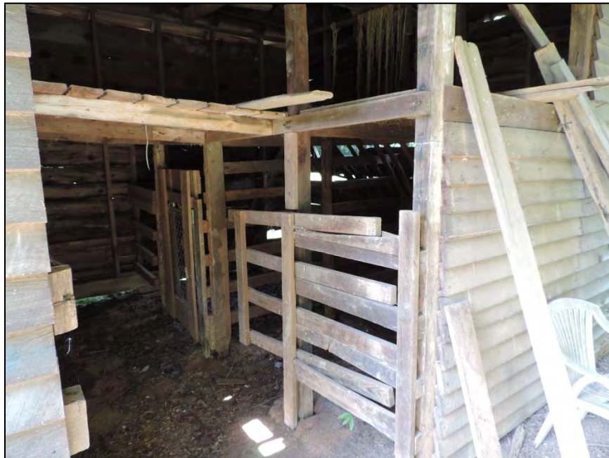
Figure 58: Suggs House, interior of outbuilding located to rear of house
