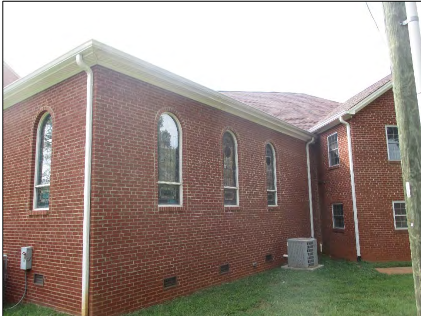
Figure 10: Center Baptist Church, facing northwest to side elevation
