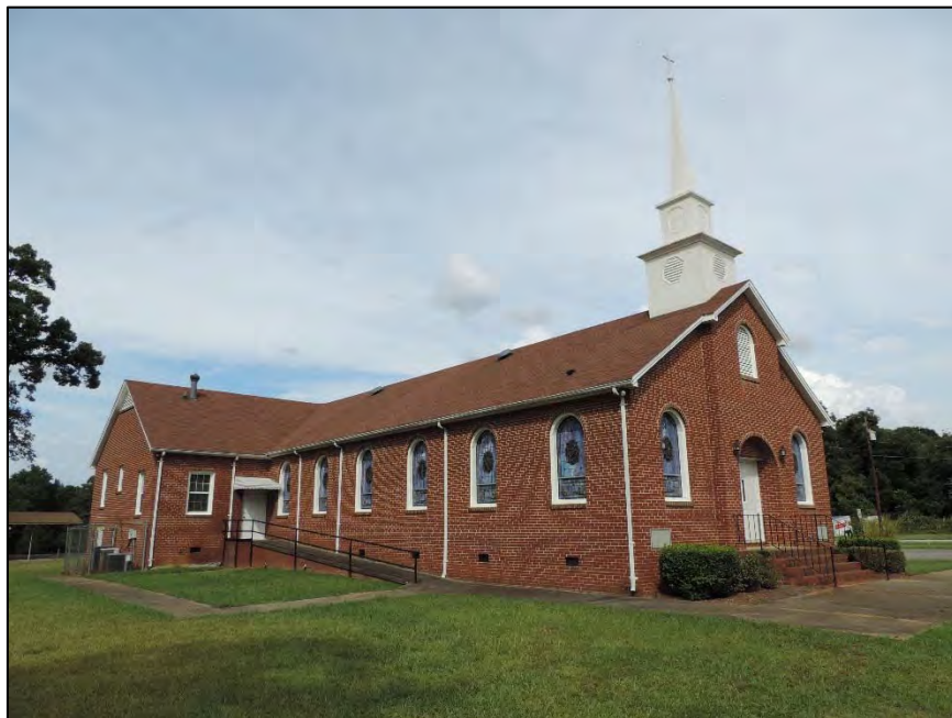
Figure 28: Facing northeast to Neely's Grove Church façade and northwest side elevation
