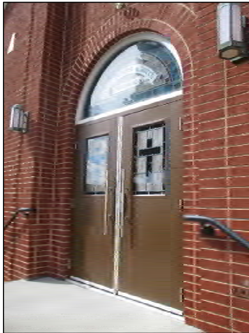
Figure 8: Center Baptist Church, entrance detail
