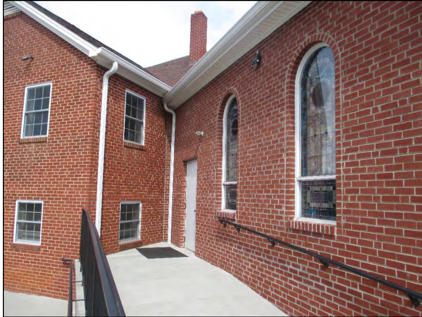
Figure 15: Center Baptist Church, facing northeast along handicap ramp
