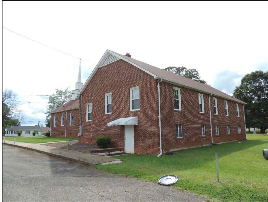
Figure 32: Neely's Grove Church, facing southwest to southeast side elevation and rear elevation
