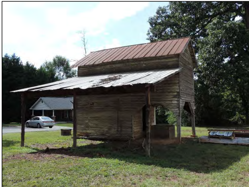
Figure 54: Suggs House, facing northwest to two-story outbuilding
