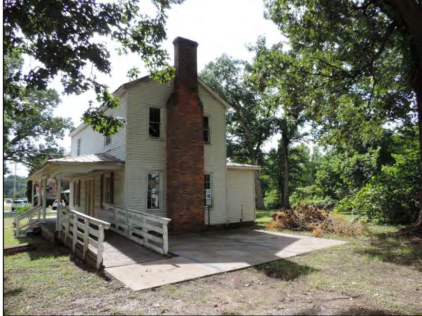
Figure 47: Suggs House, facing northwest to east side elevation
