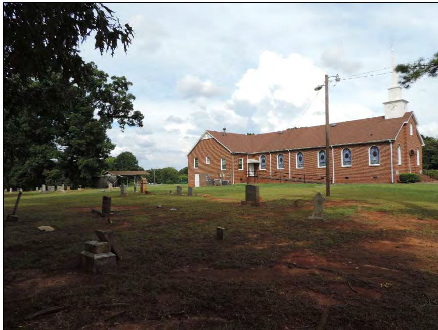
Figure 34: Neely's Grove Church, facing northeast to cemetery (Neely's Grove Church in background)
