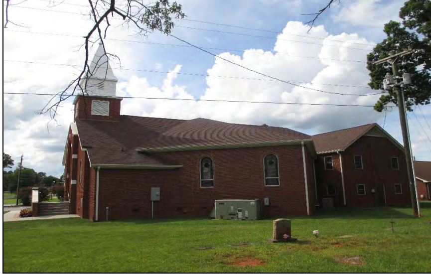
Figure 9: Center Baptist Church, facing northwest to side elevation
