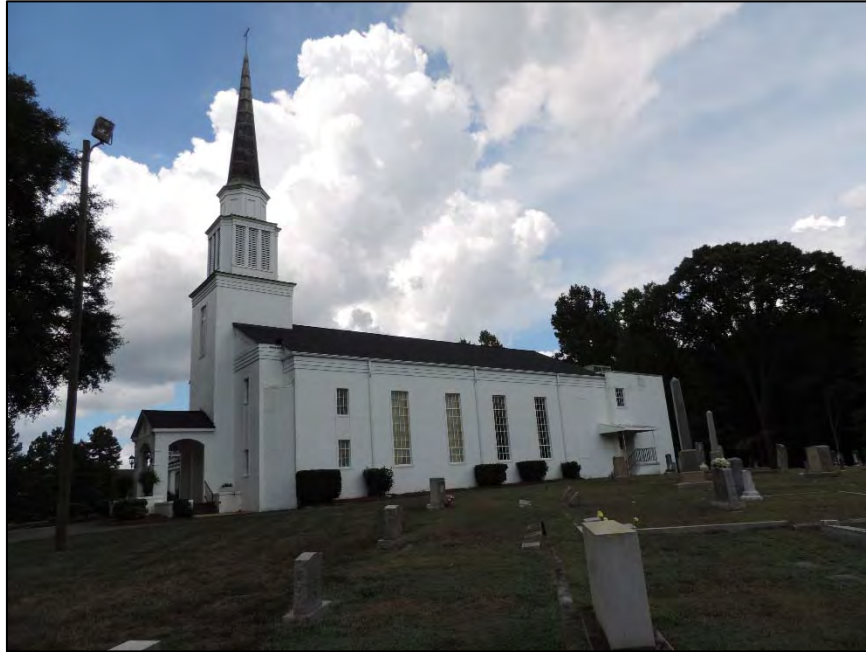
Figure 67: New Hope Presbyterian Church, facing north to south side elevation
