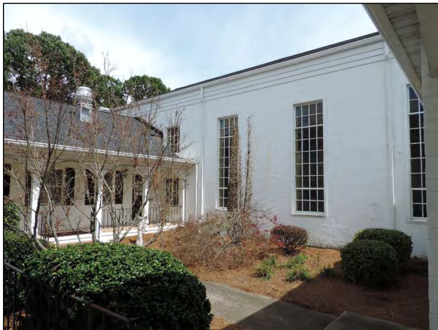
Figure 70: New Hope Presbyterian Church, facing southeast to north side elevation of church
