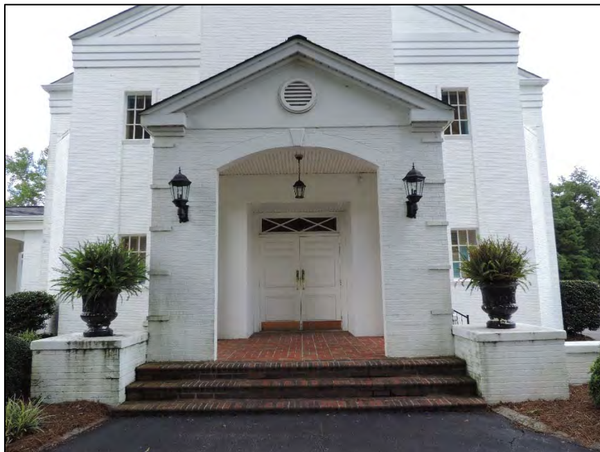
Figure 66: New Hope Presbyterian Church, entrance detail
