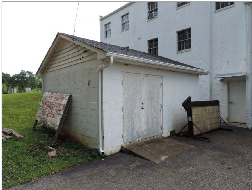
Figure 80: New Hope Presbyterian Church, facing southwest to storage building
