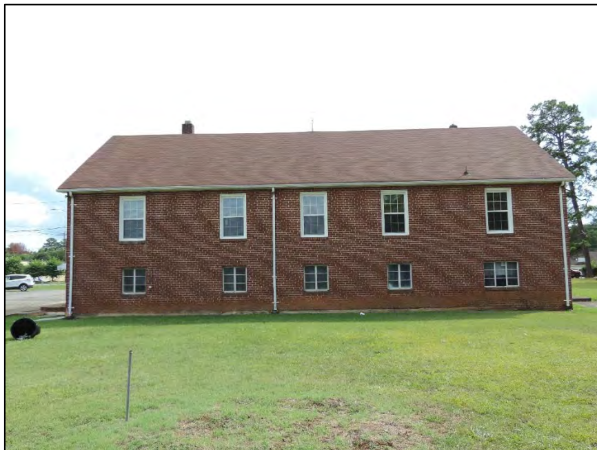
Figure 31: Neely's Grove Church, facing southwest to rear elevation
